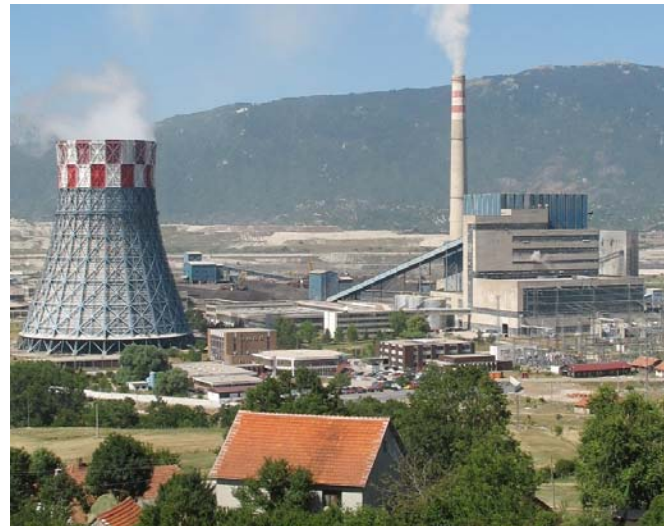
Existing Gacko facility (300 MW)
