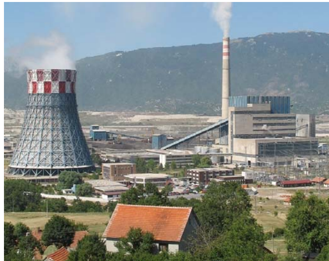
Existing Gacko facility (300 MW)
